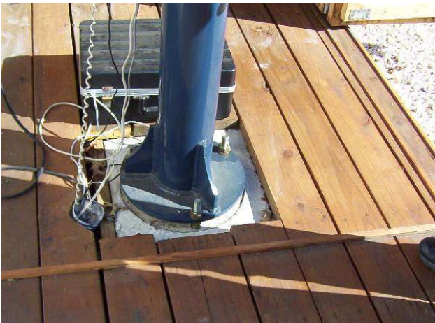
Detail of Concrete Pier
